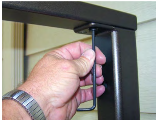
Figure 19: Tighten all screws and fasteners.
