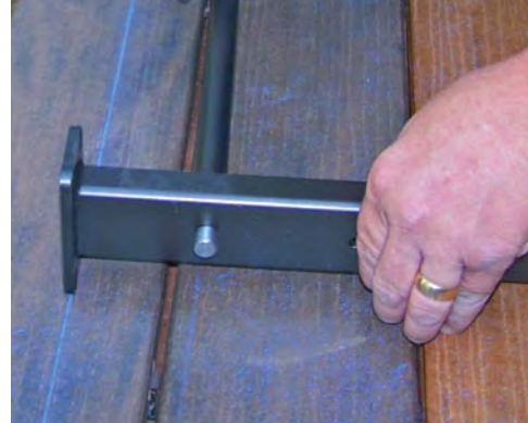
Figure 9: Install the spreader bar.
