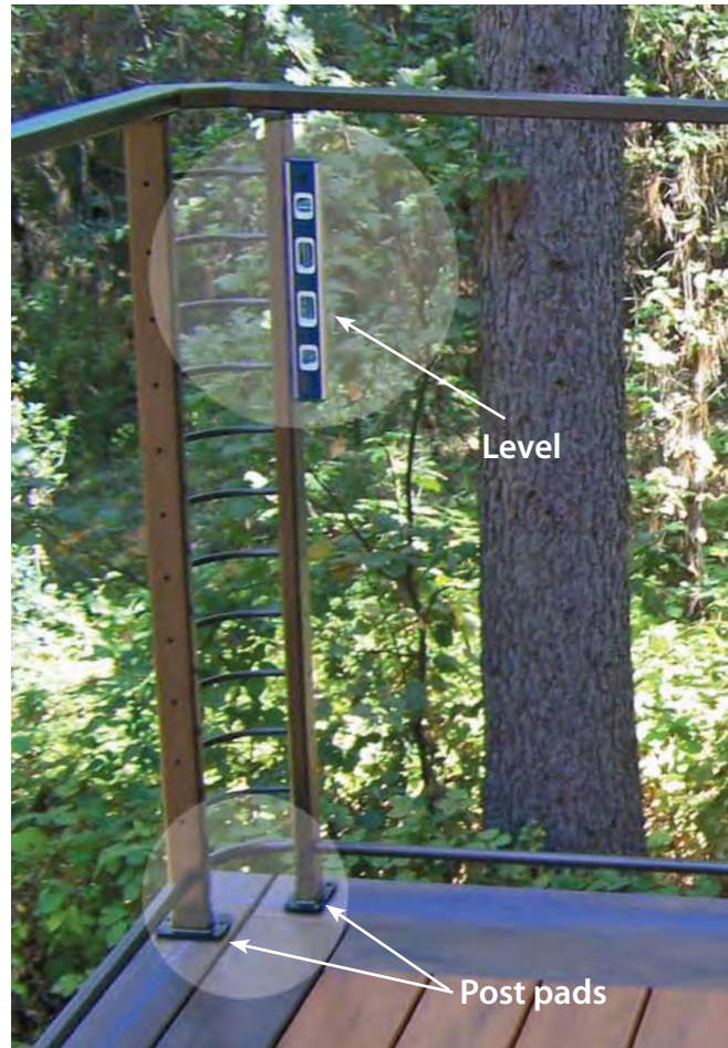
Figure 16: Use shims or washers under post pads to level the railing.
