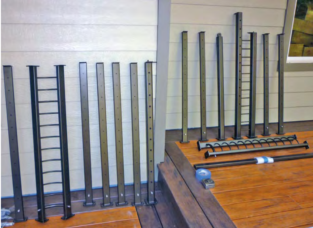
Figure 1: Separate posts, fasteners, and hardware. Check against component list provided with your order.
