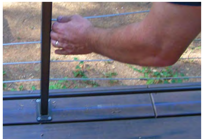
Figure 22: String cable through posts.
