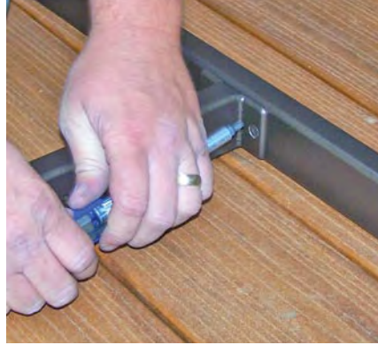
Figure 8: Attach posts to top rails.
